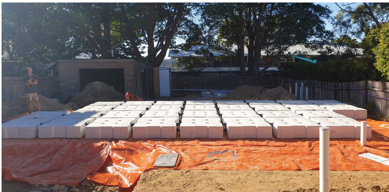
Typical Aquacomb® General Arrangement before concrete pour
